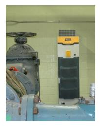
coupled to the pump shaft, requiring only a simple motor mount modification. The 200 HP AC890PX was then powered up through the existing control panel and pump sequencing logic. The available bottom power entry configuration on the AC890PX
